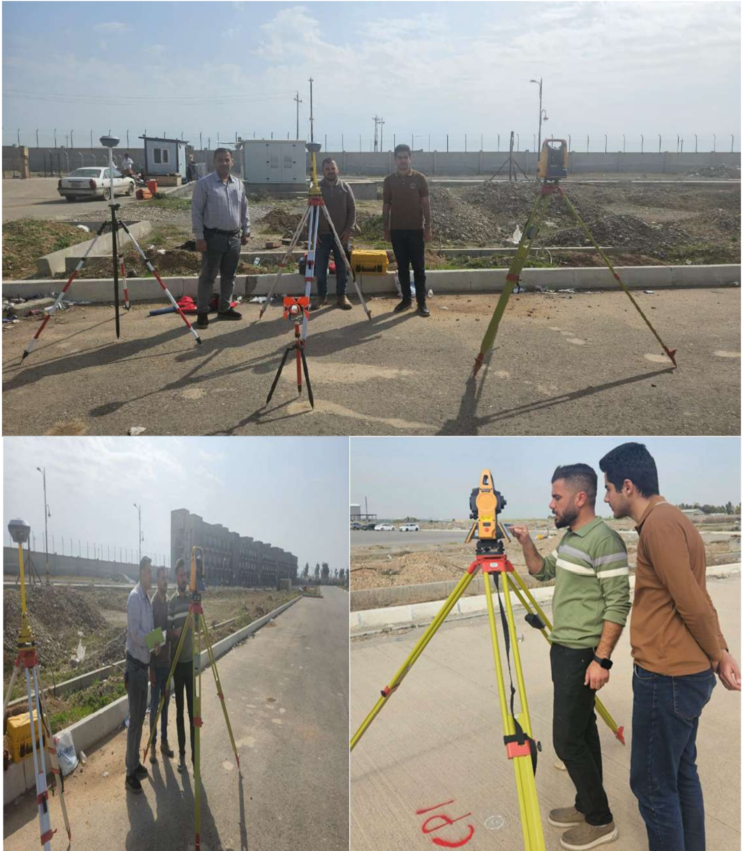
Figure 3.2: site works using total station and GNSS
