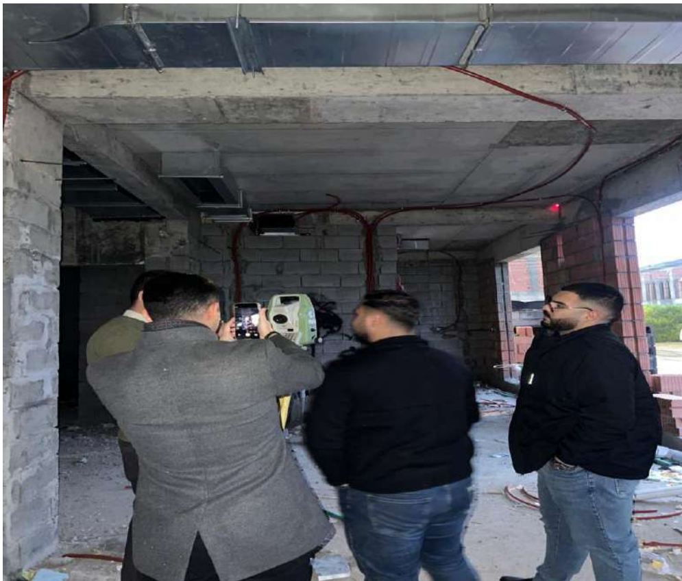
Figure (4-7) Measuring points by TS07
