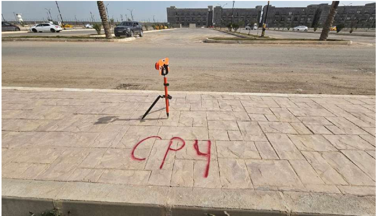
Figure 3.4: Mini Prism Setup over Established Control Point CP4
