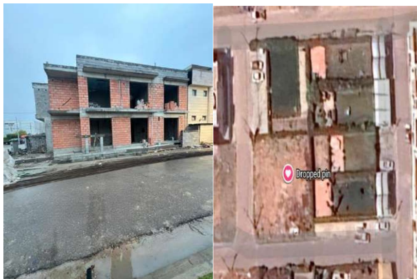
Figure 3-1 View of the building considered in the current study
