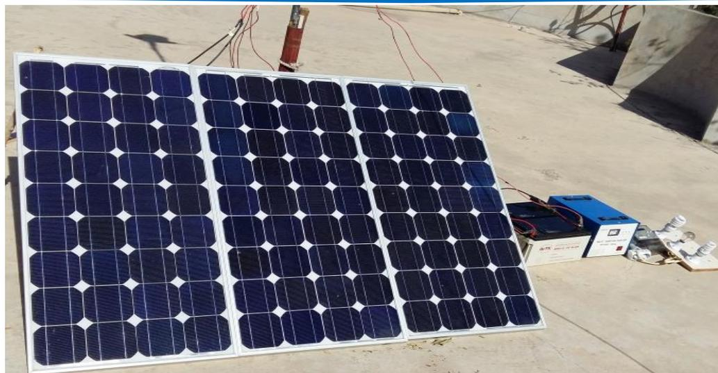
Figure 6 Energy Generation by three Solar panels of 80 W.
